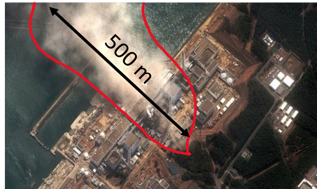
Accident at Fukushima Daiichi Nuclear Power Plant on March 11, 2011
